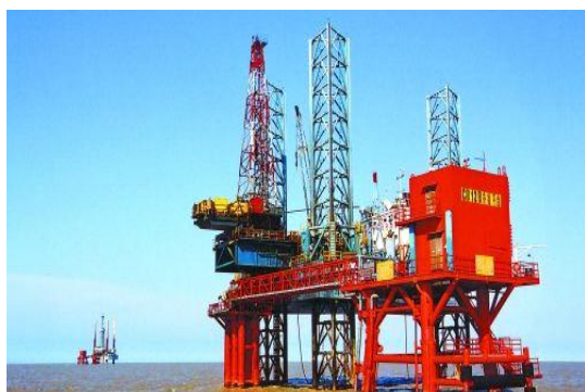
Oil field communication system
